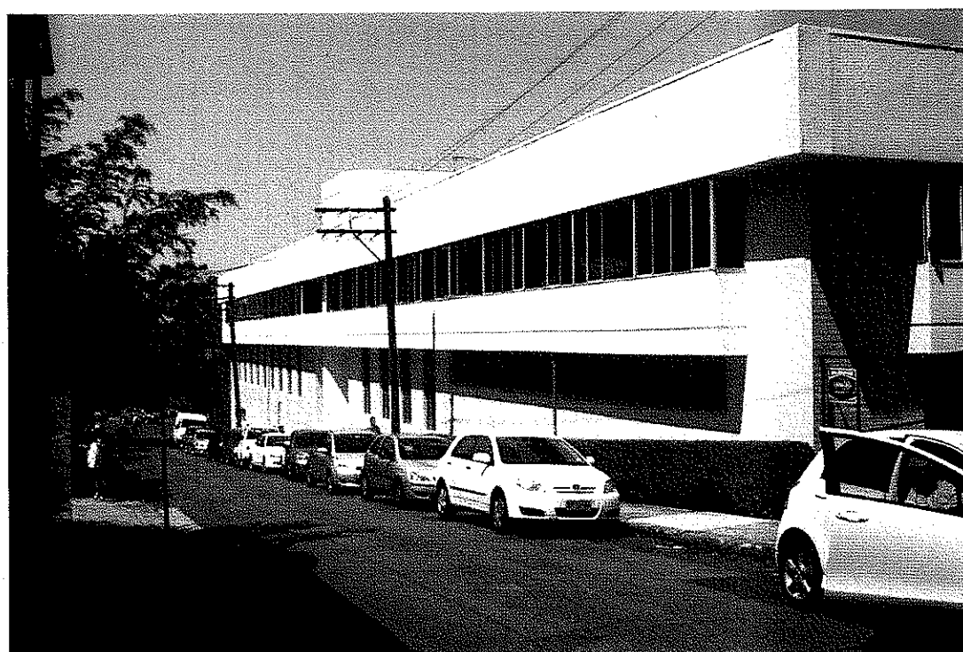
Figure 7 – Adjacent building to the east of the site (known as 162 Blues Point Road)
